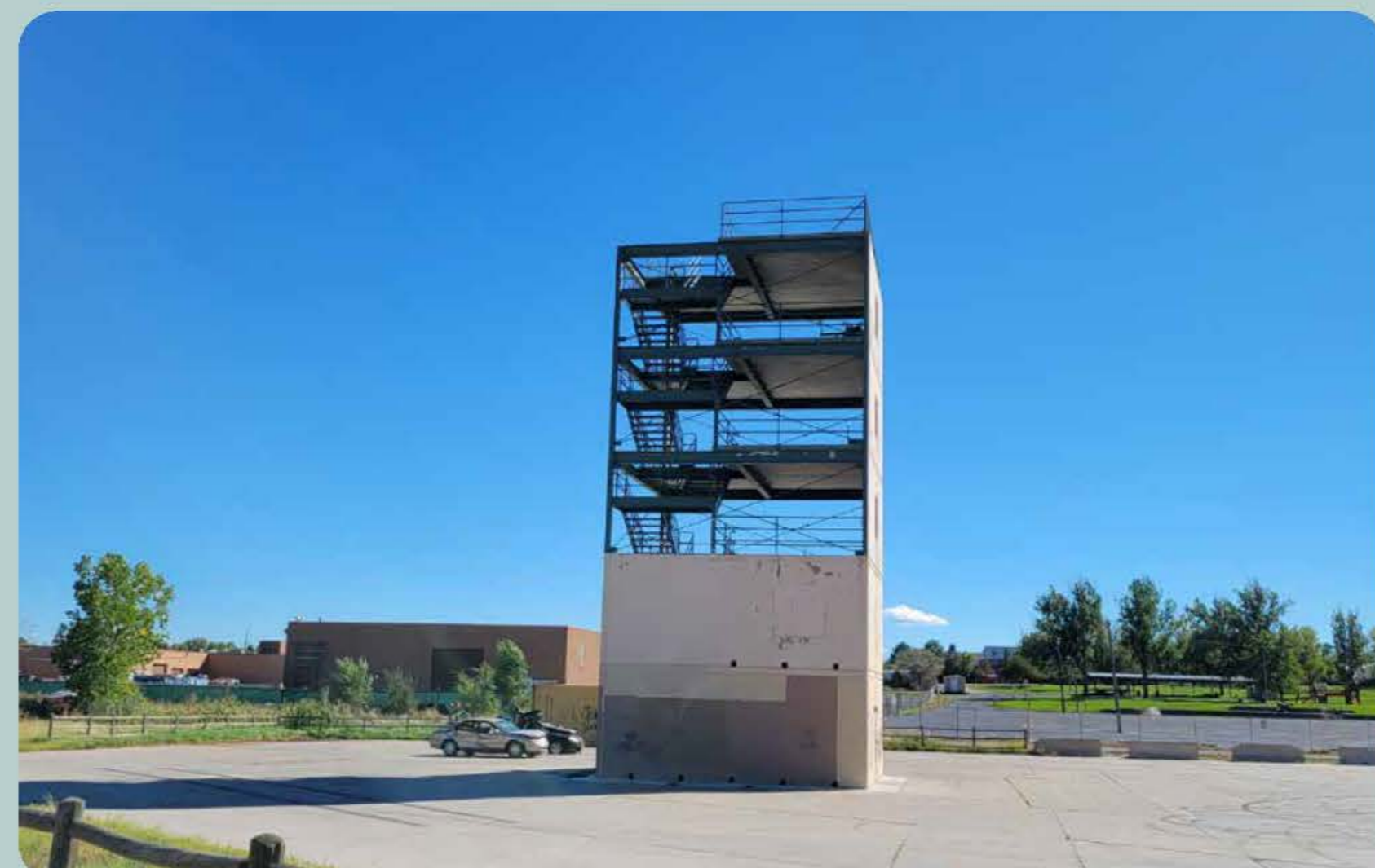
Viewing Tower (Repurpose the Fire Training Tower in the Future)
